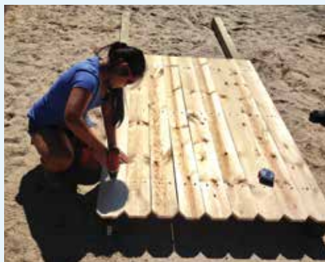
Big Sable Lighthouse Service Project
